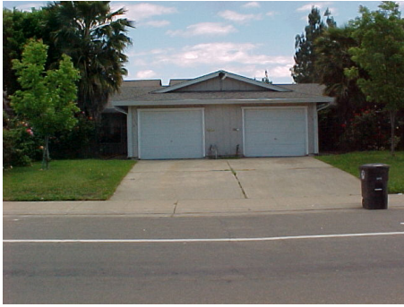
Front View of the Duplex
