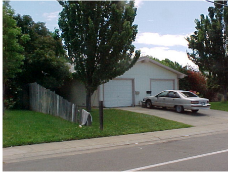
Duplex on the Right Side
